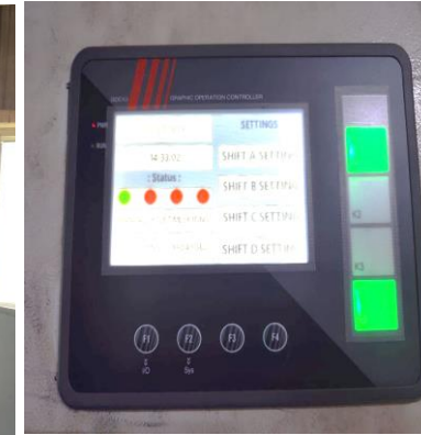
GOC fixed at dispatch area lighting load control
