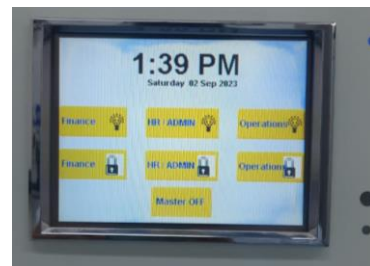
CLIPSAL OFFICE LIGHTING CONTROLLER
