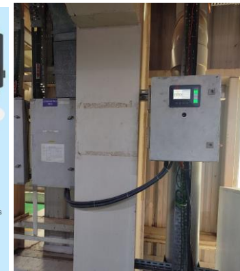
GOC fixed at dispatch area lighting load control
