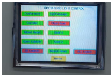
CLIPSAL OFFICE LIGHTING CONTROLLER
